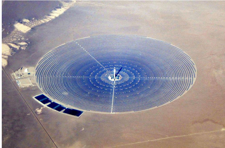
Figure 5... Concentrated Solar Power System at Crescent Dunes
