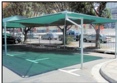
Figure 11: Permanent, galvanized steel framed canopy
