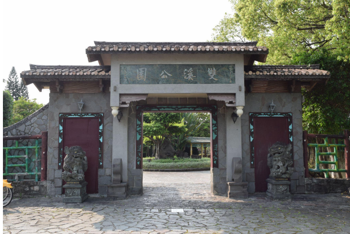
Figure 21. Entrance to Shuangxi Park
