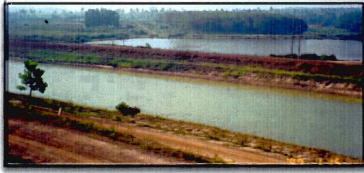
Figure 4-1: A “monkey cheek” reservoir beside the canal stores water during the dry season.
