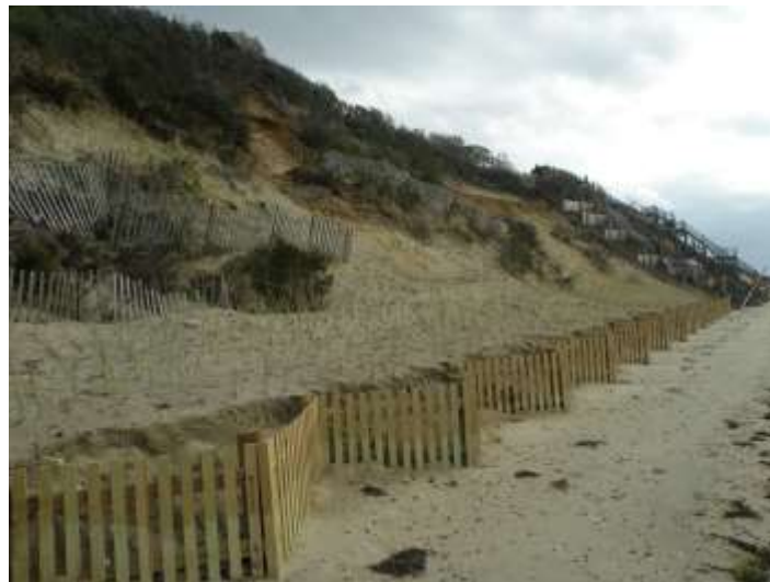
Figure 29: Zig-zag Fence, Beach Nourishment, Beach Grass, Pocomo Road Nantucket
