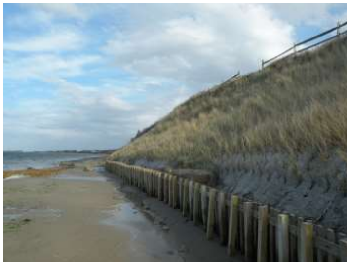
Figure 30: Linear Fence, Beach Grass Plantings, Jute Mesh, Coskata Course Way Nantucket
