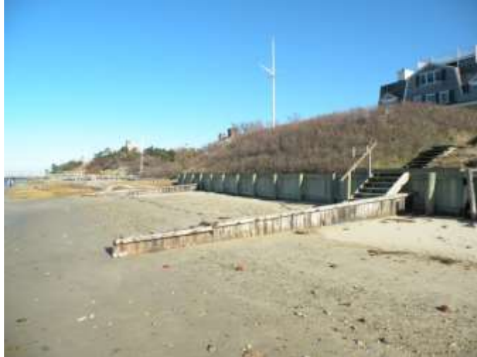
Figure 20: Timber Groins Along Shimmo Pond Road, Nantucket harbor
