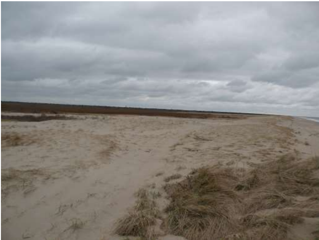
Figure 37: View of Scouring Effects from Natural Bulkhead
