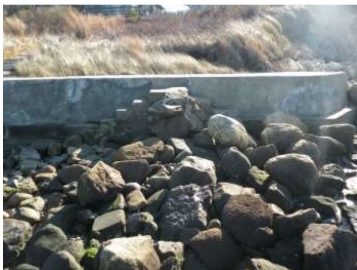
Figure 22: Close up View of Rock Groins, Quaise Road
