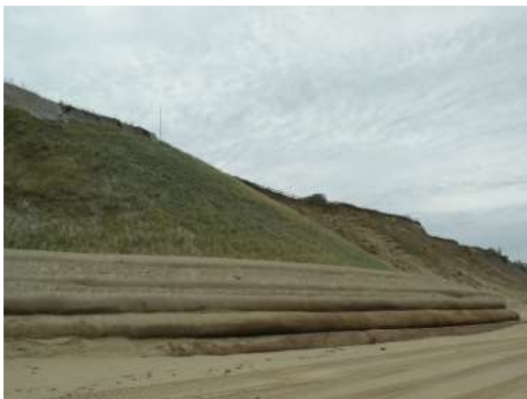
Figure 28: Jute Bags and Beach Grass, Siasconset Bluff Nantucket
