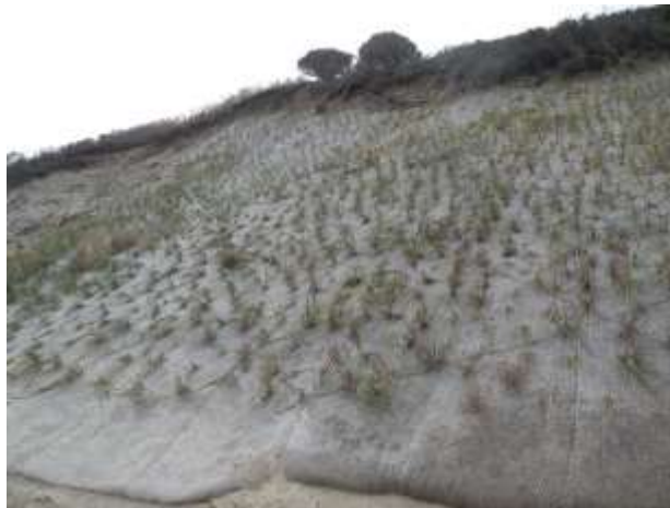
Figure8: Beach Grass with Jute Mesh, Siasconset Bluff Nantucket
