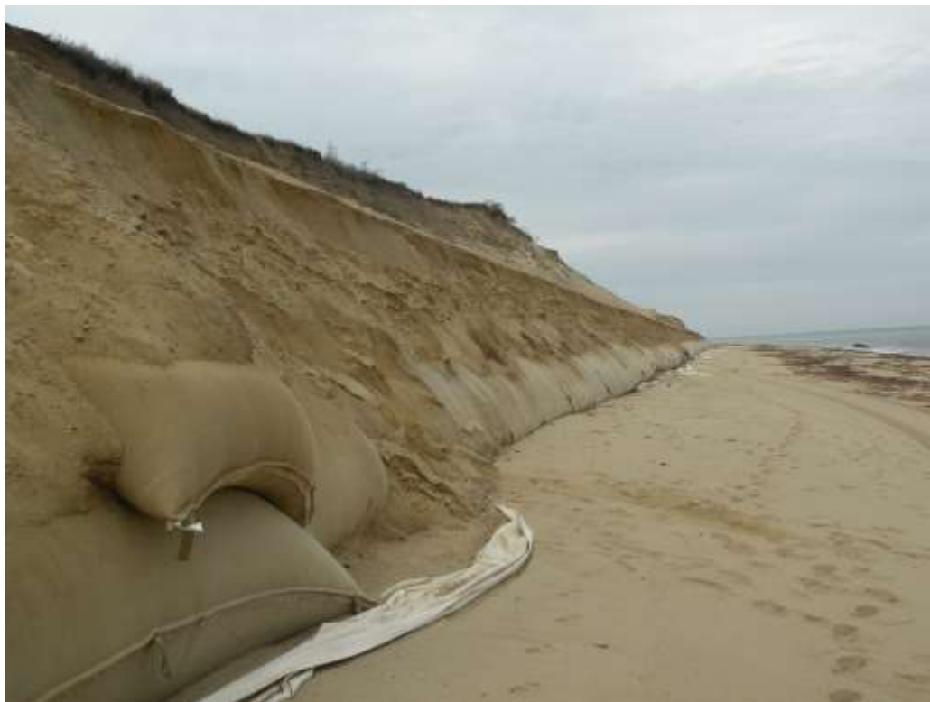
Figure 10: Geotextile Tubes, Siasconset Bluff Nantucket
