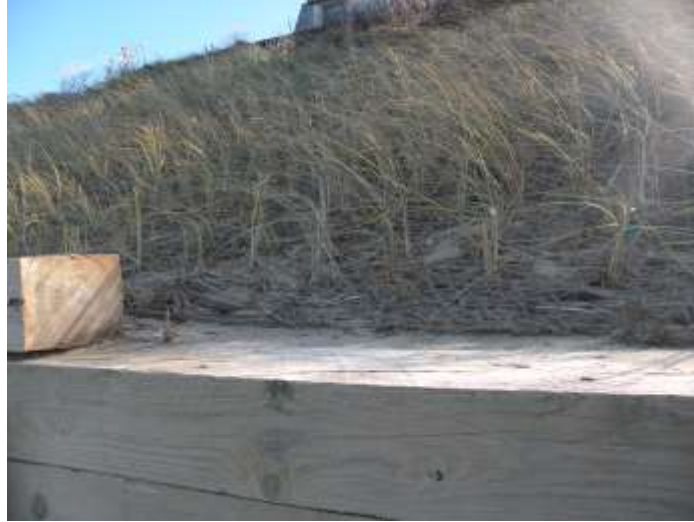
Figure 31: Wooden Bulkhead with Beach Grass and Jute Mesh, Quaise Road Nantucket
