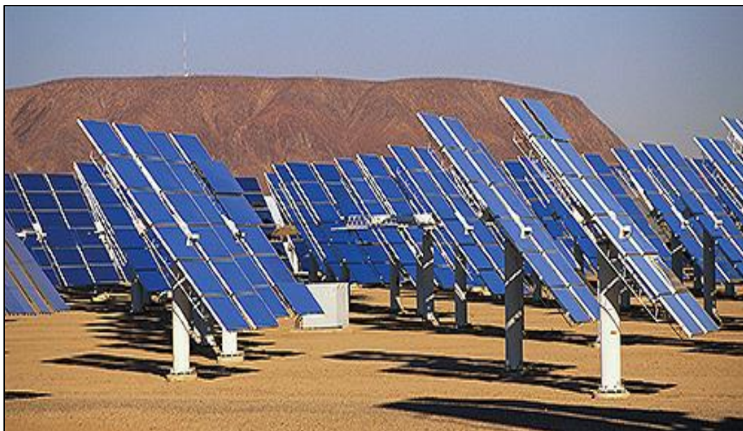
Figure 17 - Multiple PV panels mounted on the ground [22]
