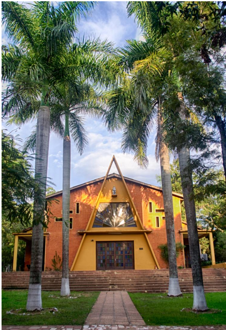
Figure 6. One of several buildings on the Escuela Agrícola campus, a retired chapel
