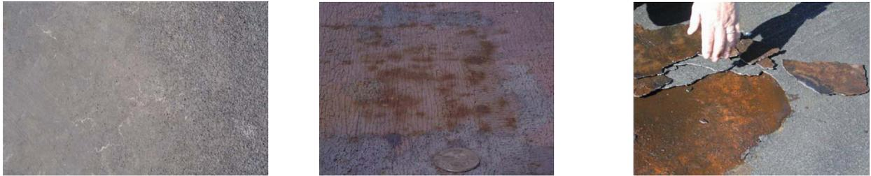
Figure 1: Traditional Non-Skid, Wear (left), Corrosion (middle), Failure (right)
