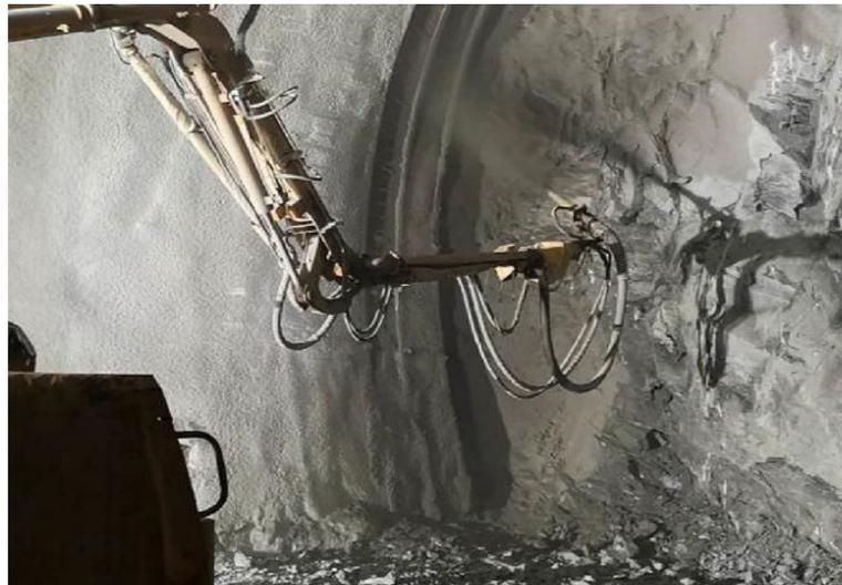
(c) Shotcrete coverage operation in tunnel construction.
