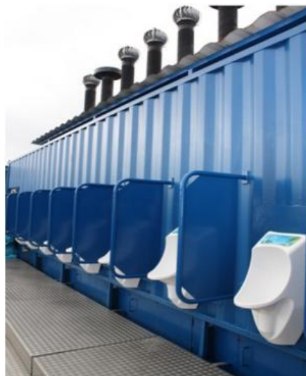
Figure 19. Urinal side of MobiSan: 12 waterless men's urinals (Quayle, 2012)
