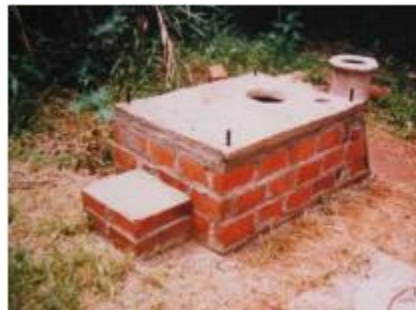
Figure 11. Front View of Vault with Toilet Slab Placed on Top (Morgan, 2007)
