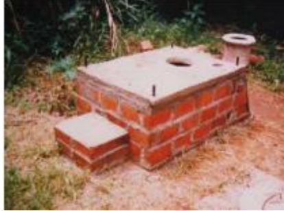
Figure 40. Front View of Vault with Toilet Slab Placed on Top (Morgan, 2007)
