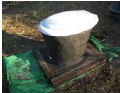
Figure 57. Completely Cemented Pedestal Curing (Morgan, 2007)
