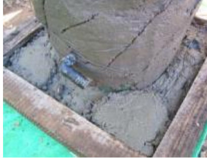
Figure 56. Wire Added for Reinforcement (Morgan, 2007)
