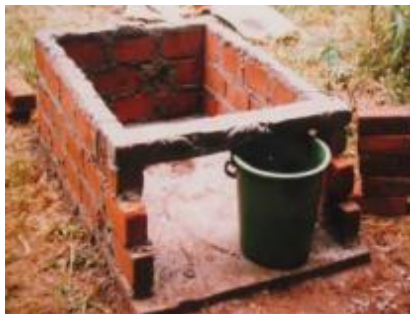
Figure 38. Vault with Concrete Lintel above 20 Litre Bucket (Morgan, 2007)
