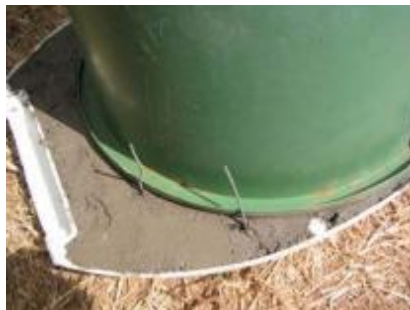
Figure 52. Bent Wire around Toilet Seat (Morgan, 2007)
