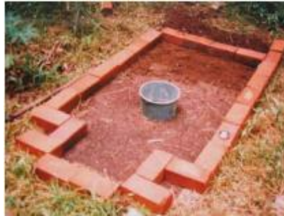
Figure 35. Brick Mould for Concrete Slab (Morgan, 2007)
