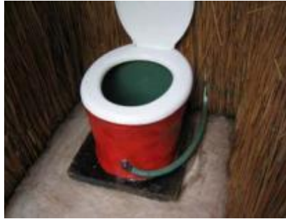
Figure 63. Installed UDDT on Slab within Straw Superstructure (Morgan, 2007)
