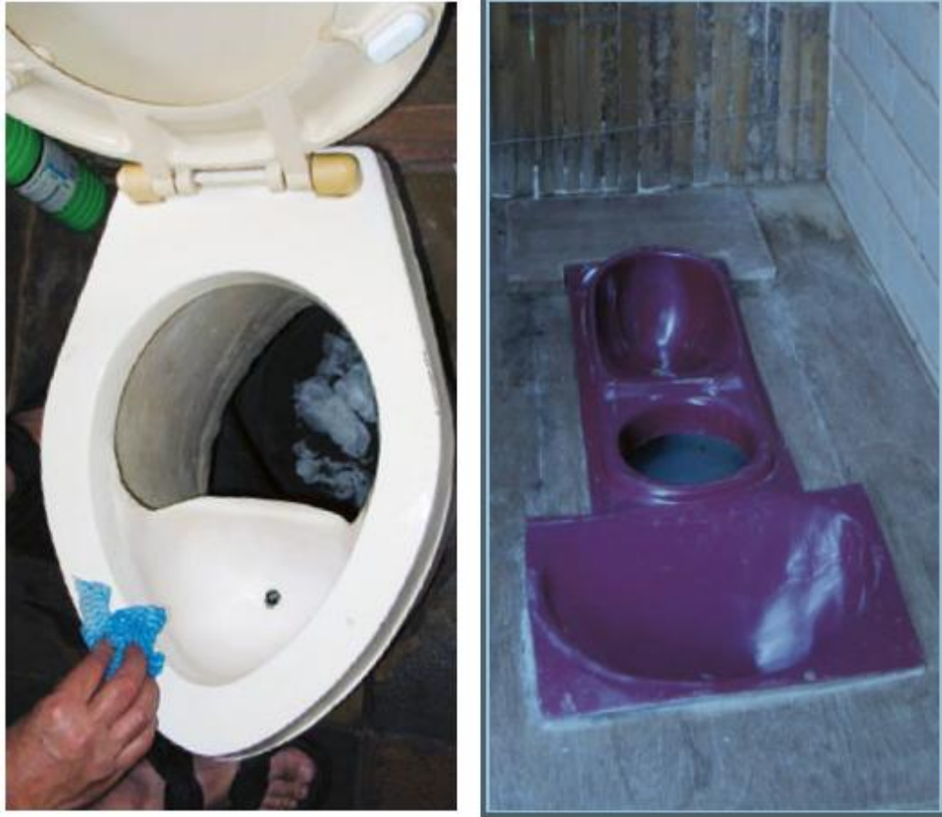
Figure 2. Left: Indoor UDDT (pedestal type) in Johannesburg, South Africa (Münch, 2006 from Münch and Winker, 2011). Right: UDDT Squatting Pan in Bangalore, India, with three holes: the area in the front is for anal washing; middle is for feces and back is for urine (Schafer, 2008 from Münch and Winker, 2011).
