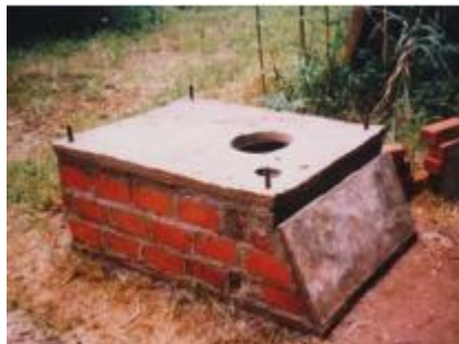
Figure 12. View from Behind Vault Showing Slanted Concrete Access Slab (Morgan, 2007)
