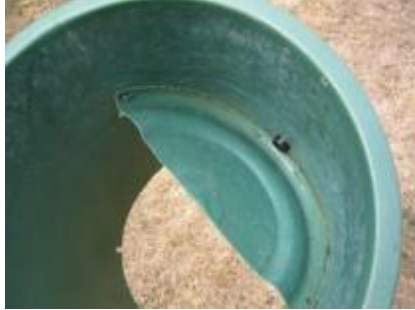
Figure 47. Inside View of the Fitted Pipe Bend (Morgan, 2007)
