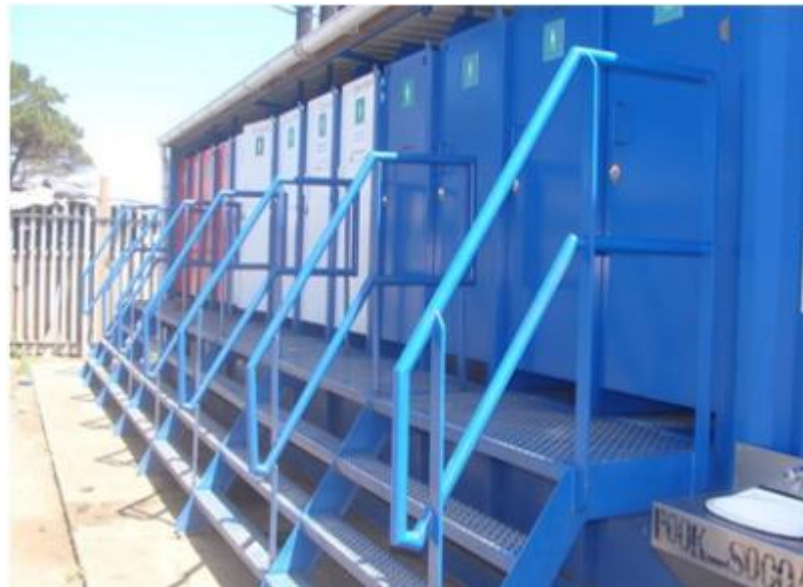
Figure 18. Toilet side of MobiSan: 13 UDDTs separated by gender and age (Quayle, 2012)
