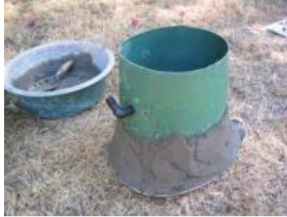
Figure 53. Concrete Added Half-way up Bucket (Morgan, 2007)
