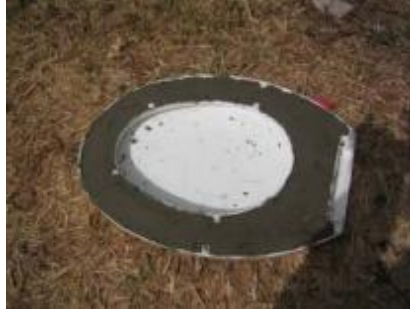
Figure 50. Concrete Added to the Toilet Seat (Morgan, 2007)
