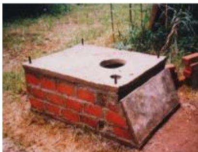
Figure 39. Fitting Vault Access Slab (Morgan, 2007)
