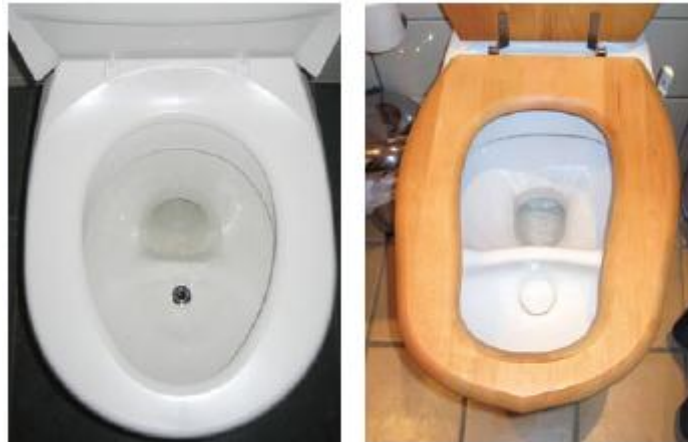
Figure 4. UD Flush Toilets. Left: Gustavsberg (in Meppel, the Netherlands). Right: Dubbletten (in Stockholm, Sweden) (Münch, 2007 from Münch and Winker, 2011).
