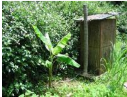
Figure 64. Urine Pipe Led to Banana Tree (Morgan, 2007)
