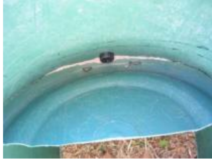
Figure 59. Urine Diverter Sealed from Top (Morgan, 2007)
