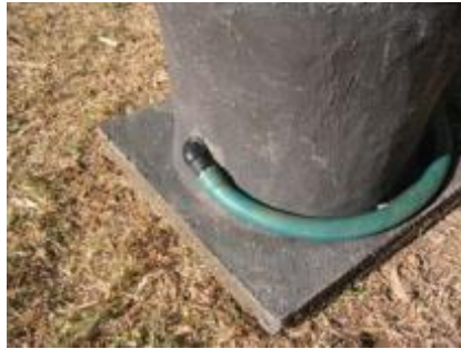
Figure 60. Attached Urine Pipe (Morgan, 2007)
