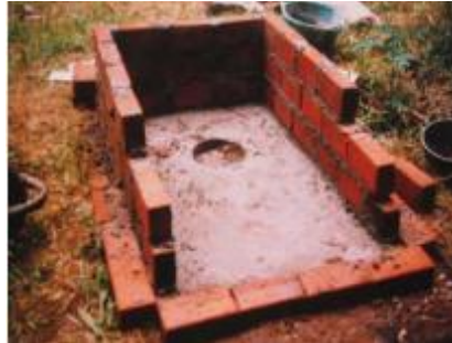
Figure 37. Vault Using Bricks on Their Edge (Morgan, 2007)
