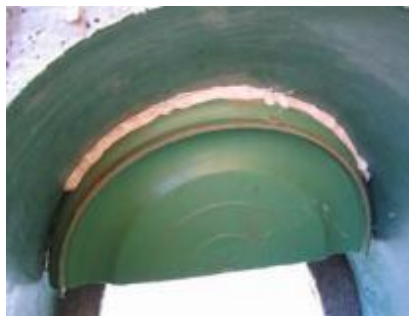
Figure 58. Urine Diverter Sealed from Bottom (Morgan, 2007)
