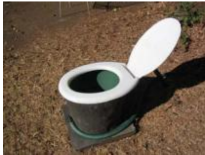
Figure 61. Urine Pipe Led to Rear of Toilet (Morgan, 2007)
