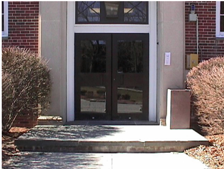
Figure G.1: Glass Door, Metal Frame
