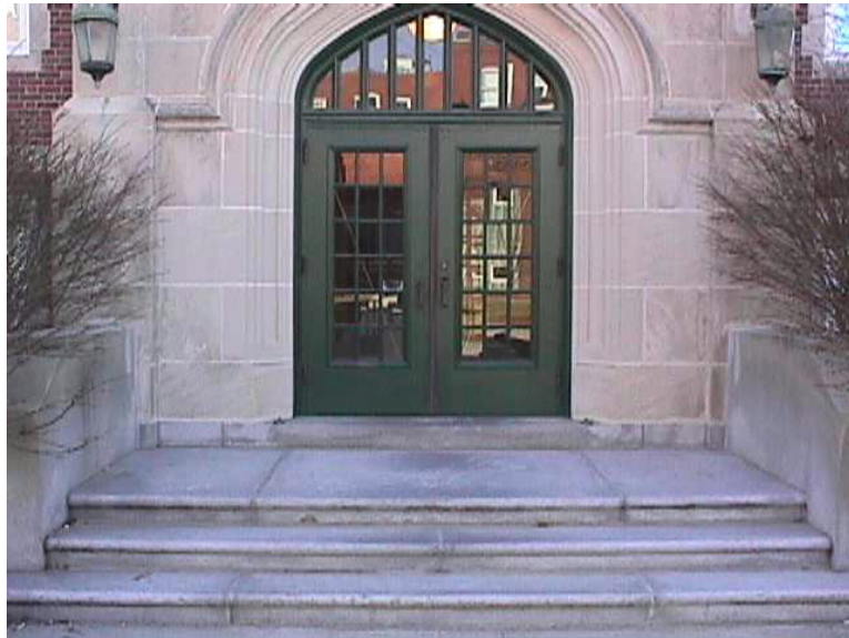
Figure G.8: Wood Door, Wood Frame, Glazed
