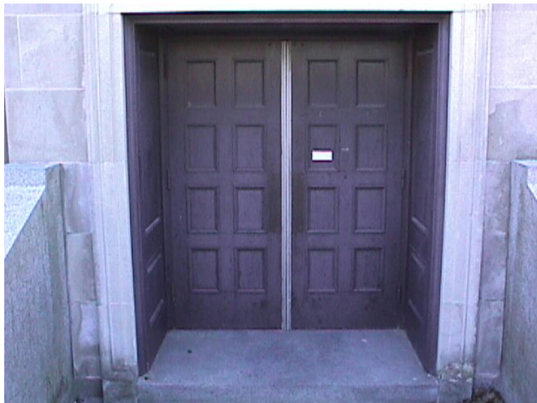
Figure G.4: Wood Door, Wood Frame, Panels
