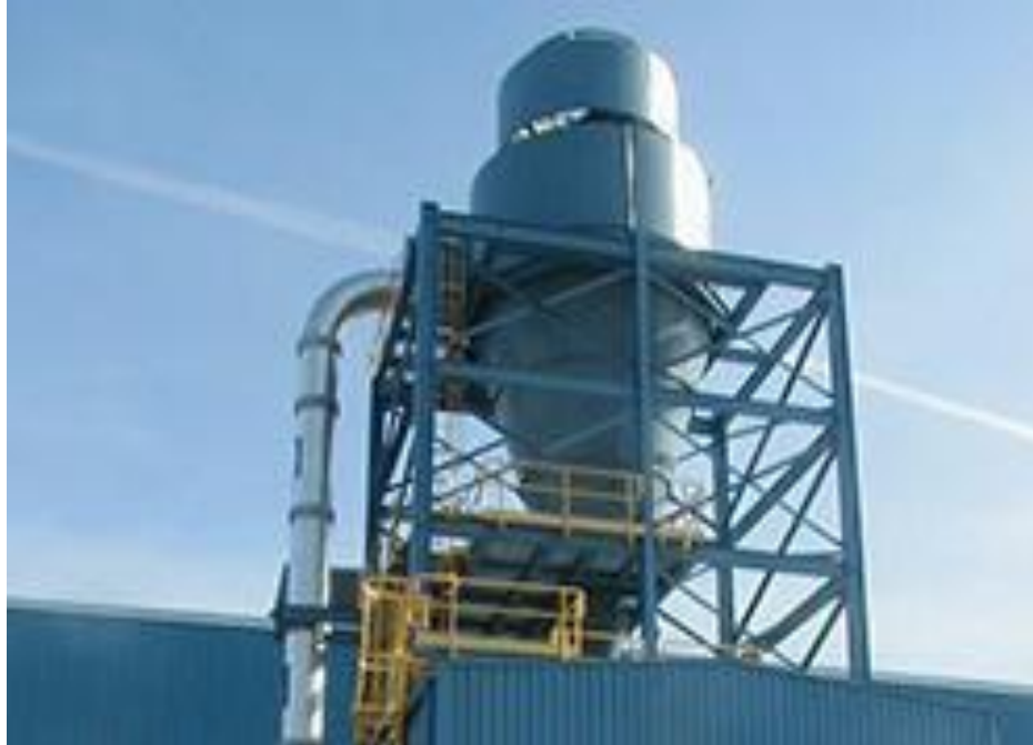
Fig. 5: A Cyclone Fed by a Vacuum Tube [13].
