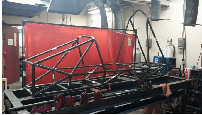
Figure 83 Frame Fully Tacked
