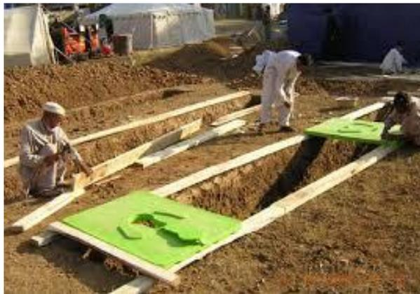
**Figure 30:** Showing the construction of a trench (Excreta Management, (n.d.))
