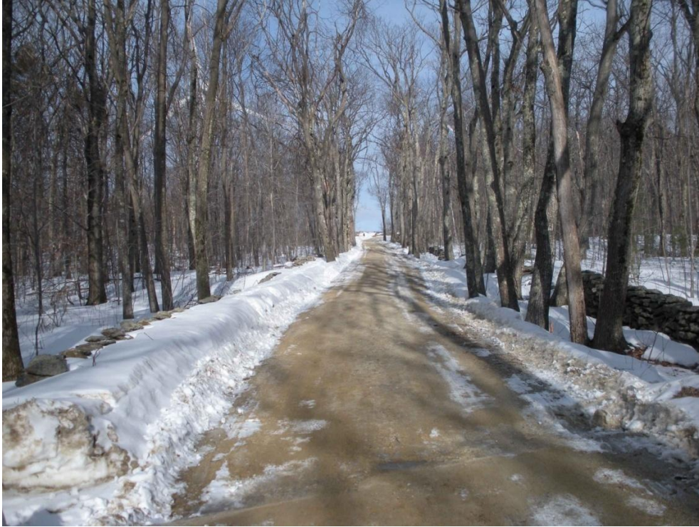
Figure 41 - Imagine showing a waterbar on Princeton's access road
