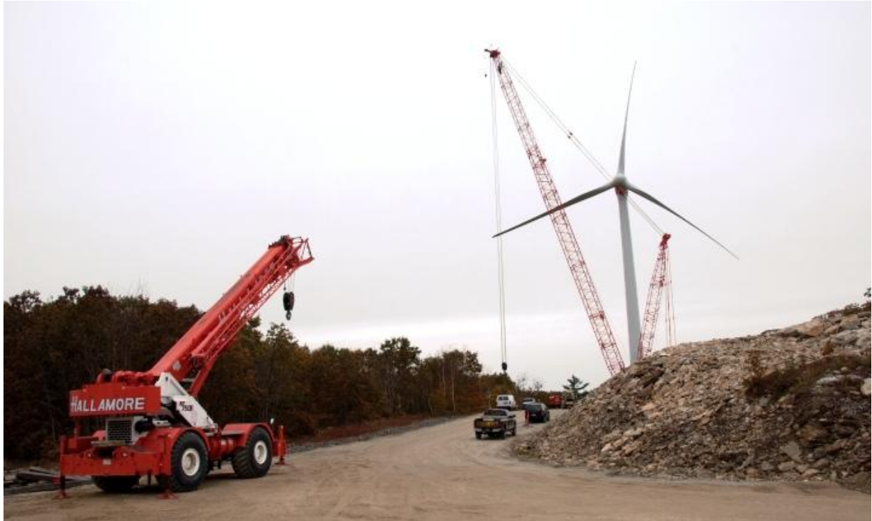
Figure 11: Princeton access road on staging area
