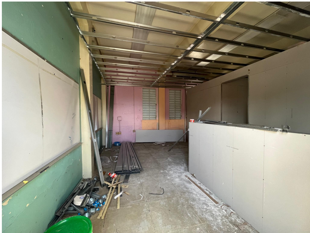
Figure 14: Photo of Classroom in Cubuy-Lomas Center during Renovation Process
