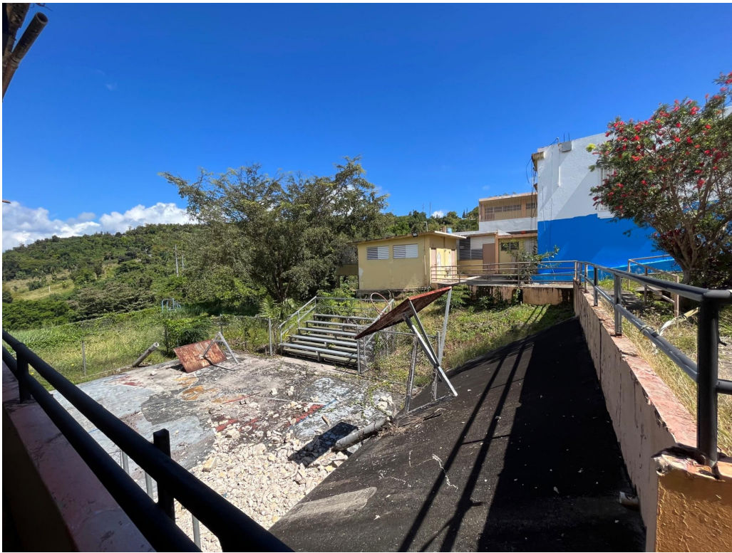
Figure 13: Photo of Recess Area at Cubuy-Lomas Center
