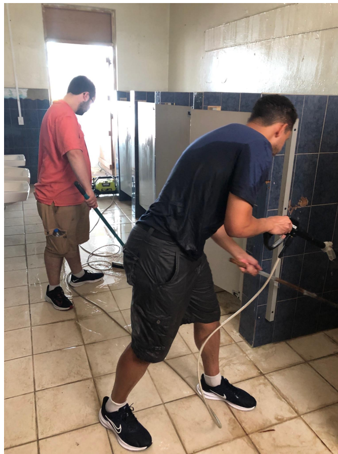
Figure 4: Power-Washing the Bathroom at La Goyco's Brigade
