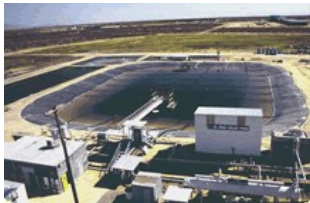
Figure 2.2 Solar pond in El Paso Texas [47]
