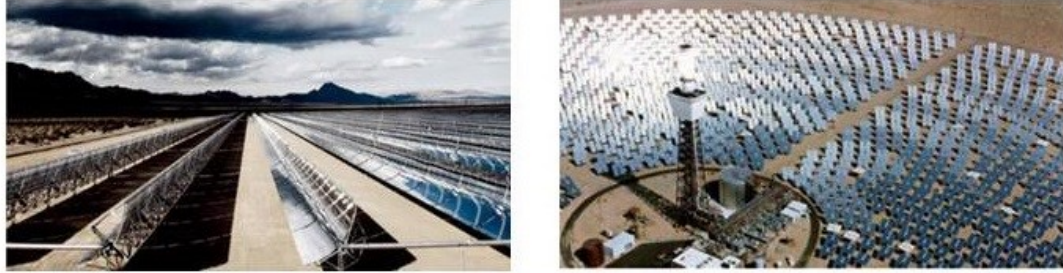
Figure 1.2 Left: line focused collector, right: point focused collector [12]
