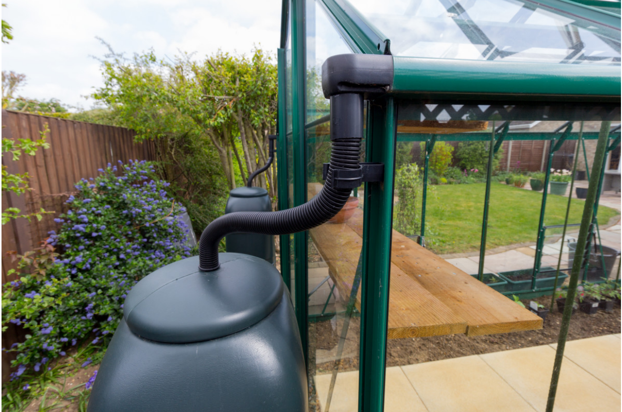
Figure 9: This image from DenGarden.com 31 shows an example of a gutter rainwater collection system that could be implemented in future greenhouse designs. The most important aspects shown are that the barrel and gutters are fully closed and opaque. This prevents the growth of algae, which are deleterious to a hydroponic system.
