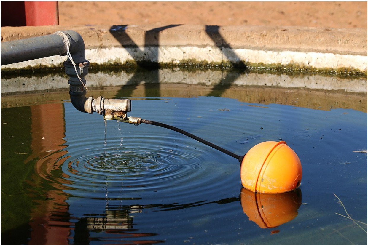
Figure 7: This is an example of a basic float switch in practice 29 .
