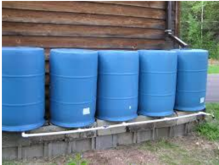
Figure 15: Multi-Barrel Harvesting System Image Source: Pinterest.com
