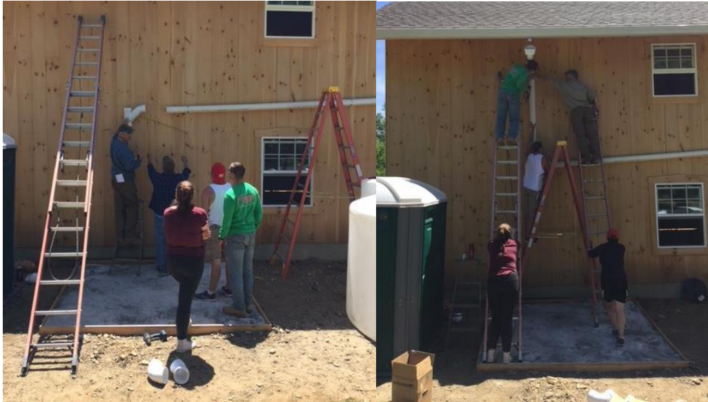
Figures 18 & 19: Construction Day 2: Finishing Collection System Image Source: Lisa Stoddard
