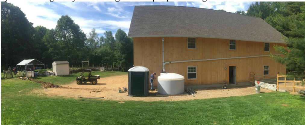
Figure 4: Completed Rainwater Catchment System Image Source: Virginia Adams
