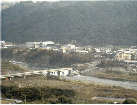
Surface faulting from the Chi-Chi earthquake destroyed the Bei Fon Bridge.
