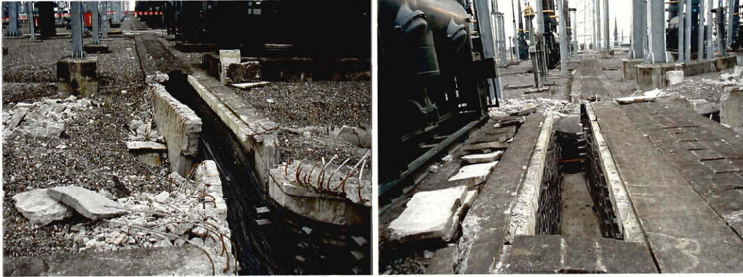
There was much delicate repair work that needed to be done.
