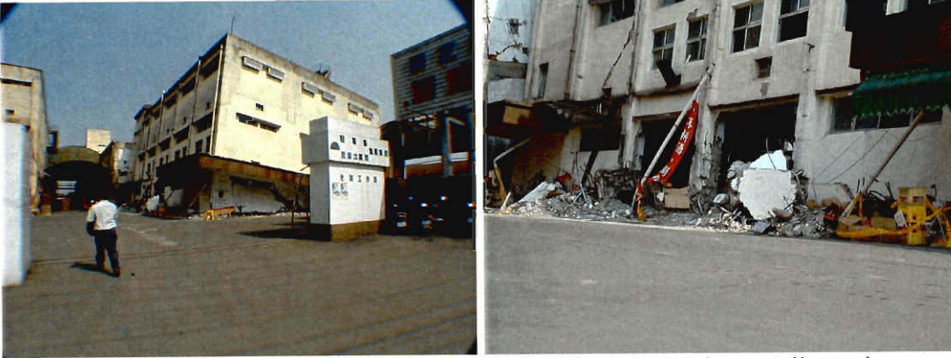
The camera was held straight; it's this building in Puli that is actually no longer upright.
