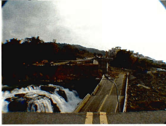
Surface faulting from the Chi-Chi earthquake destroyed the Bei Fon Bridge.
