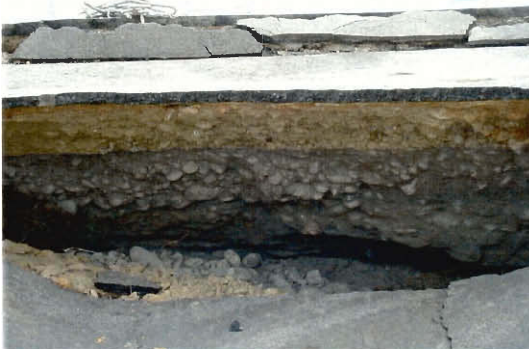
(Left) The surface deformation made the soil layers very easy to distinguish. (Right) The ground beneath railroad tracks going through the harbor collapsed.
