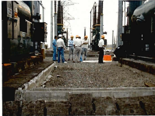
Workers consider the best ways to repair the damage done.
