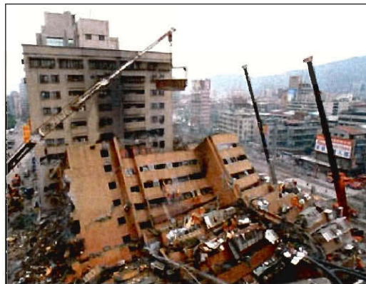
Figure 6.19 The Tunghsing Building in Taipei used to stand 12 stories high
