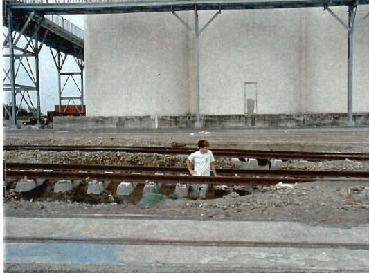
(Left) The surface deformation made the soil layers very easy to distinguish. (Right) The ground beneath railroad tracks going through the harbor collapsed.
