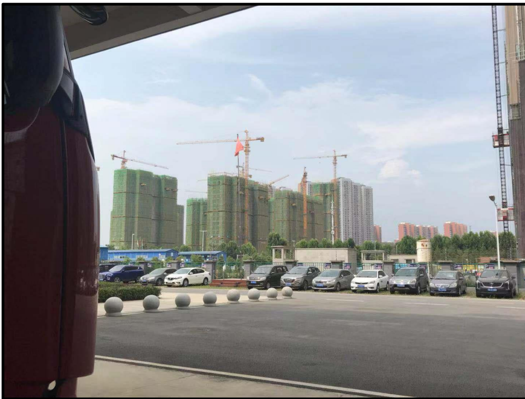
Figure 10: Construction Outside the Fire Station
