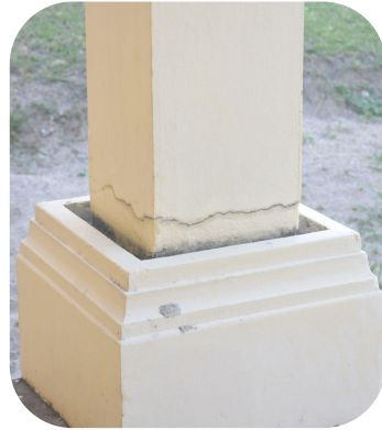
Horizontal Crack
