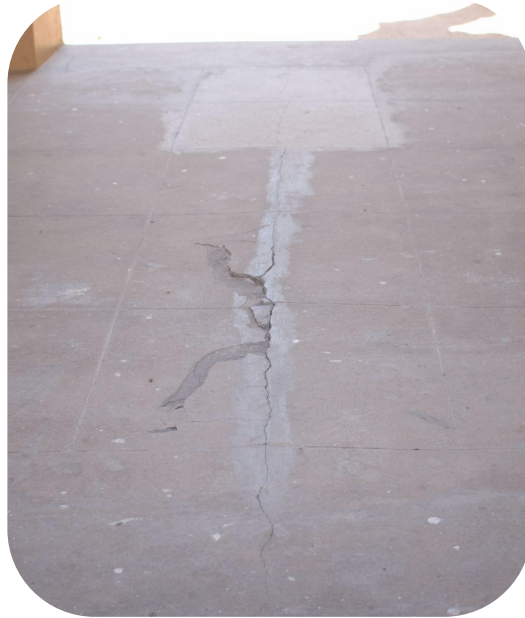
Concrete Floor Base
