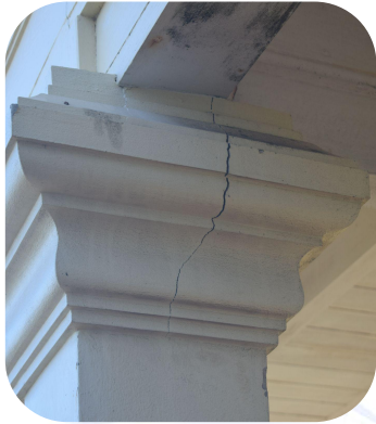
Vertical Crack
