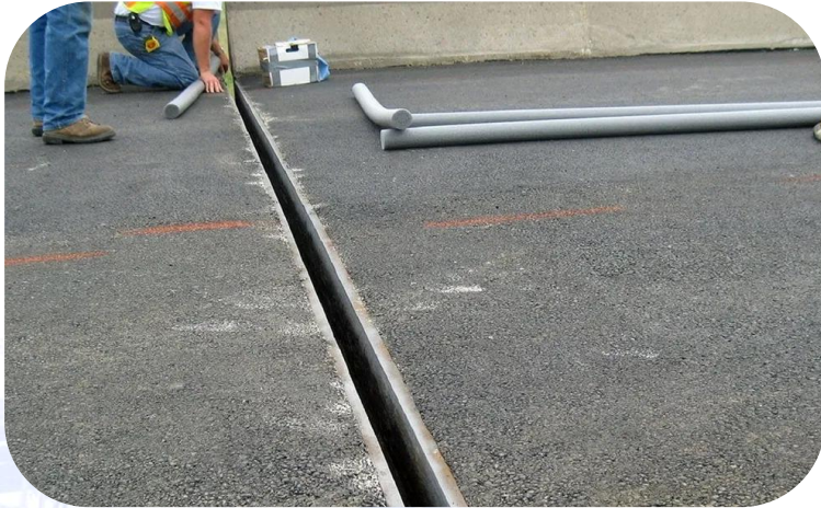
Example of Expansion Joints
