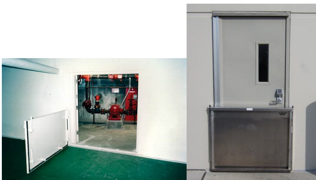
Figure 20: Hinged flood gate examples
