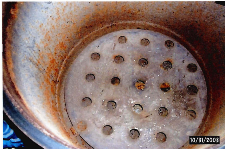
Figure 2: Interior of one of the retorts, lined with rust.
