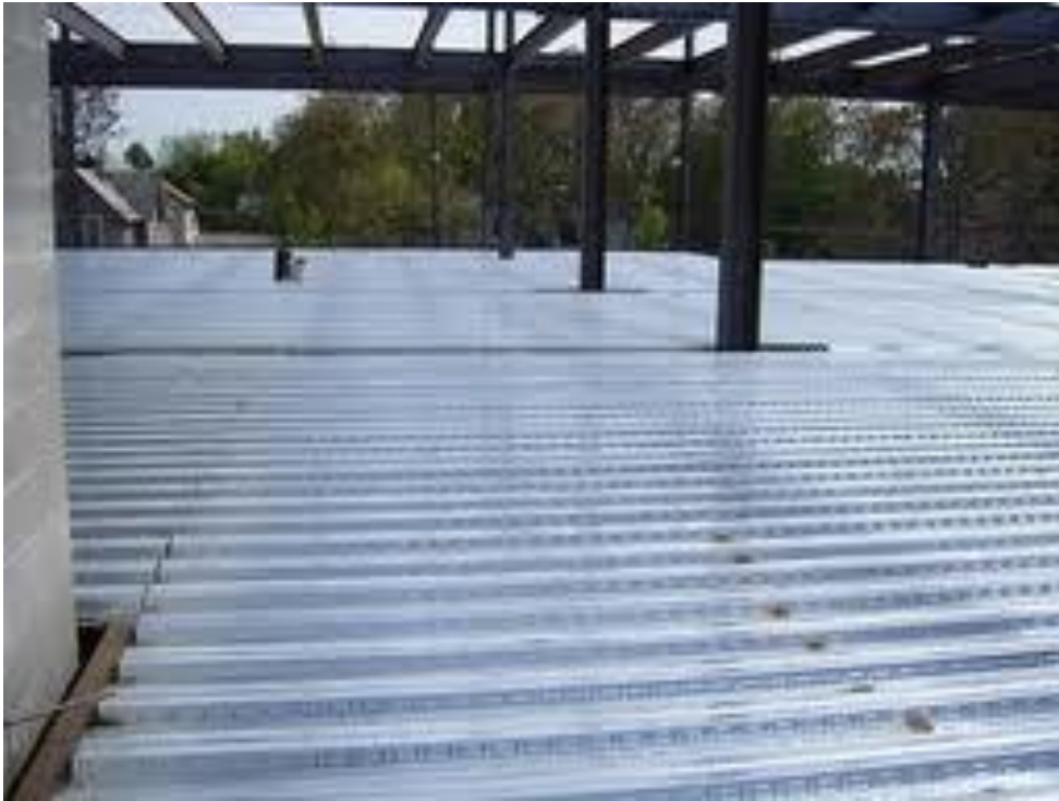
Figure 7: Steel decking before a concrete pour 5
