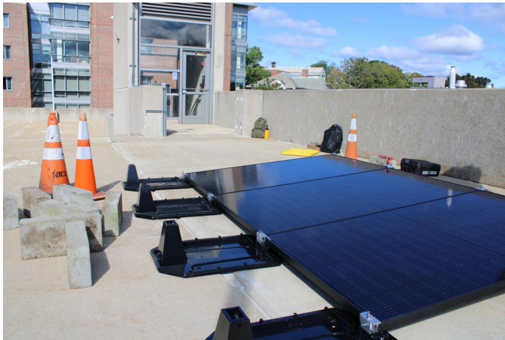
Figure 20. The PV array after the successful installation at the site.
