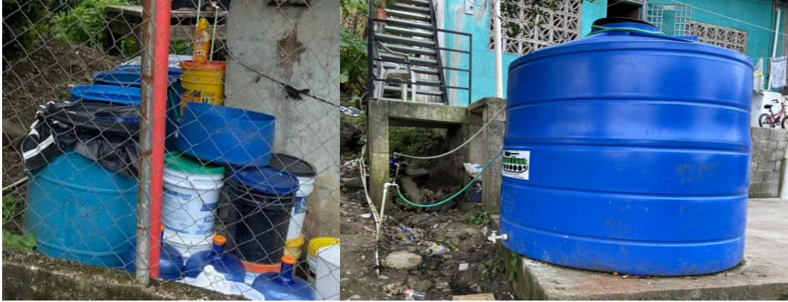
Figures 2.16-2.17. Examples of residential water storage tanks in Villa Cardenas and Valle de San Francisco where people store excess water and sometimes use their own pump systems to deliver it to their home.
