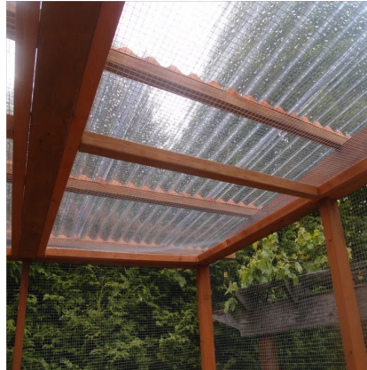
Figure 24: Example of Clear Plastic Sink Ceiling
