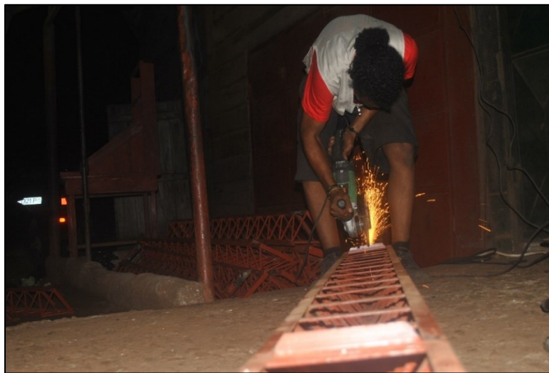
Figure 55: Worker using an angle grinder while building the AMP spacecraft (Agboglobshie Makerspace Platform, DSC_0410, 2014)
