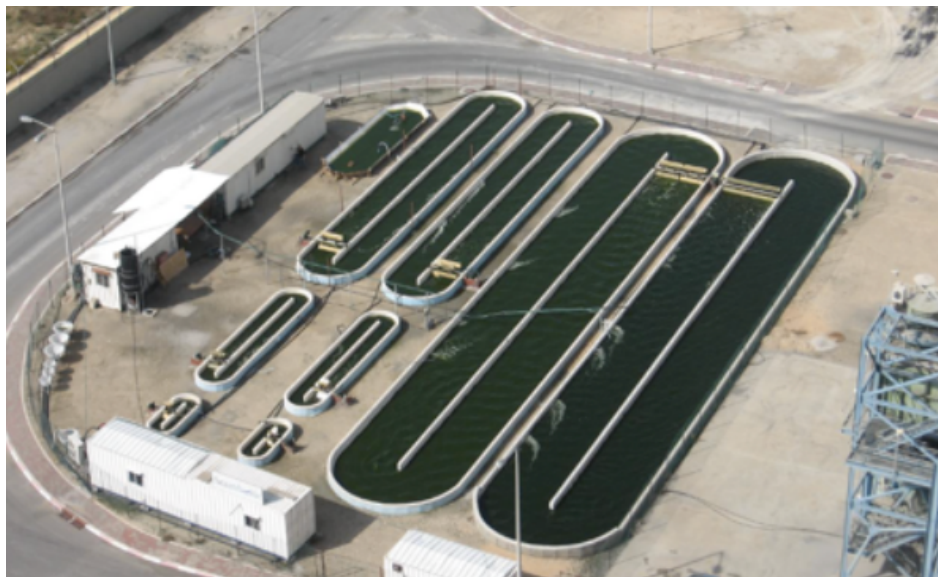
Figure 8: This is an open raceway pond (ORP) built for Seambiotic in Israel. Source: (Williams II and Pagan, 2018)
