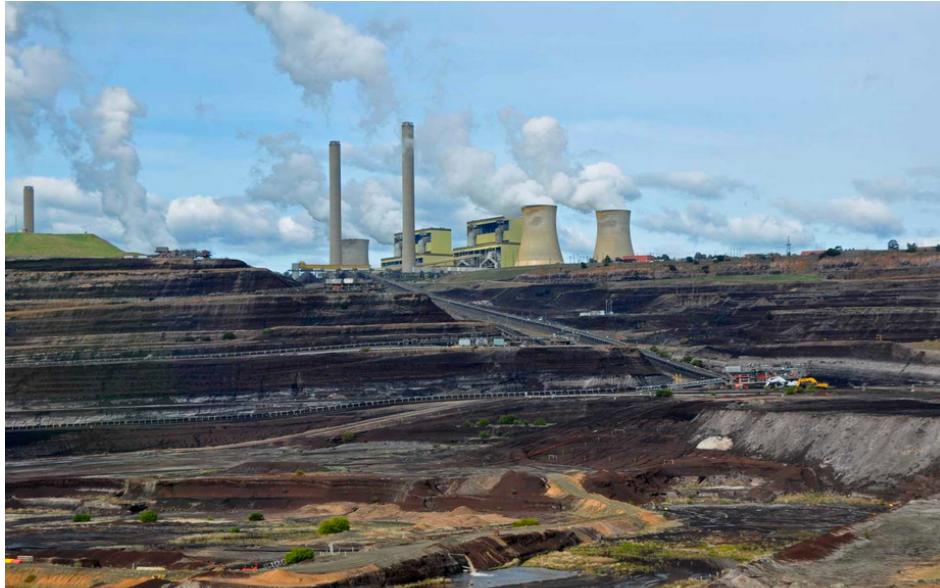
Figure 16: Hazelwood Power Plant mines.
