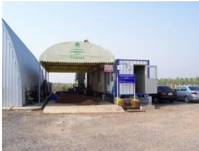
Figure 21: Reception station (left) and container for processing equipment (right).
