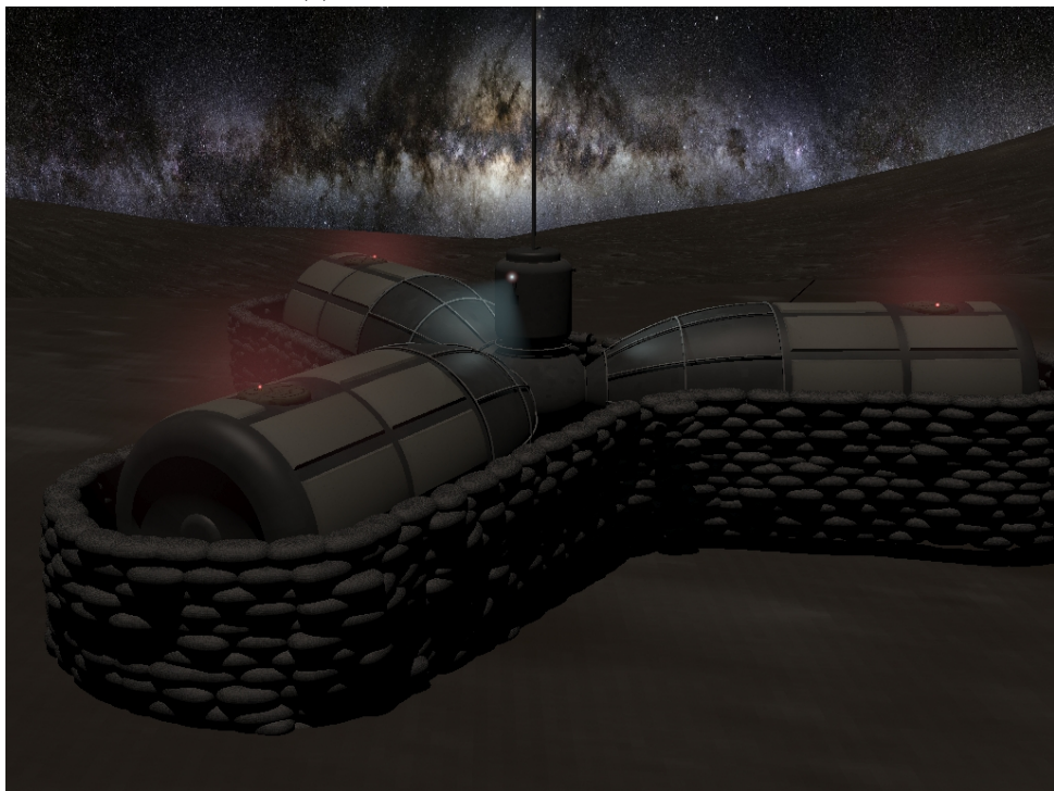
(b) Phobotian Outpost partially covered by Sandbags for Radiation Shielding
