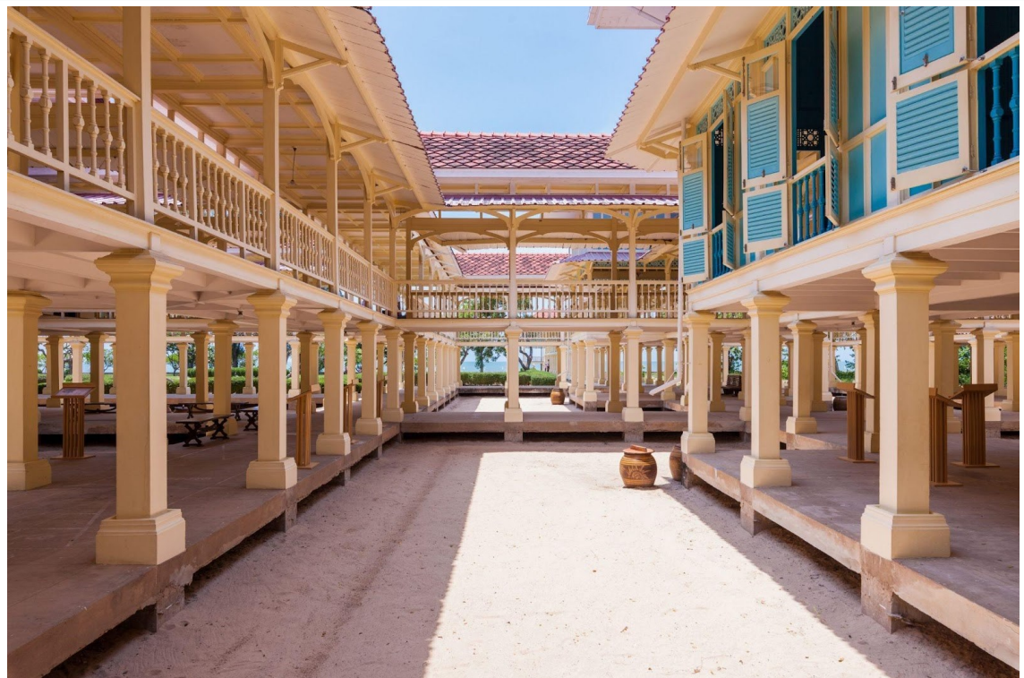
Figure 11. Photo of the Palace's Column Supported Walkways and Living Quarters 18
