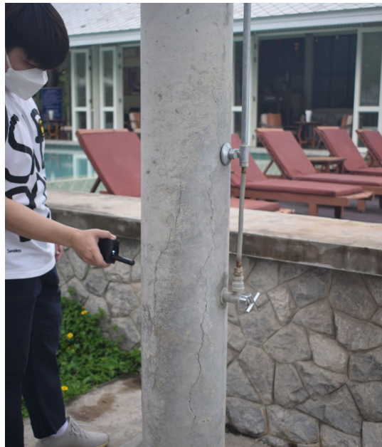
Figure 10. Metal detector instrument used to find steel reinforcement in columns
