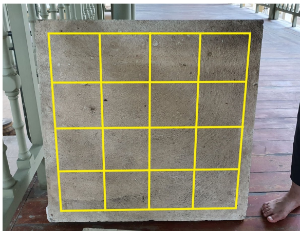
Figure 29. Steel reinforcement pattern in a ceiling panel
