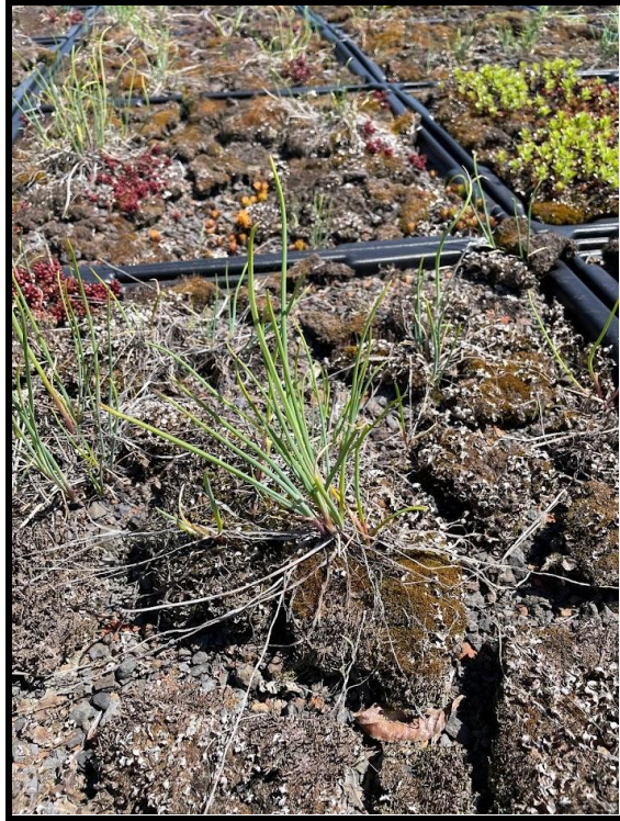
Figure 13. Chives on the East Hall green roof, April 2023
