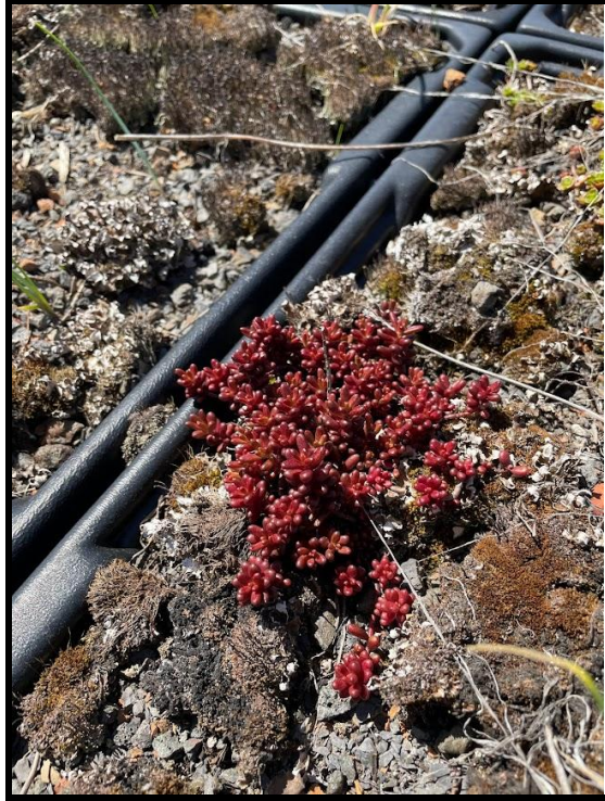
Figure 11. Red sedums on the East Hall green roof, April 2023
