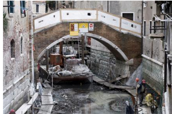
Figure 3 - A canal undergoing repairs
