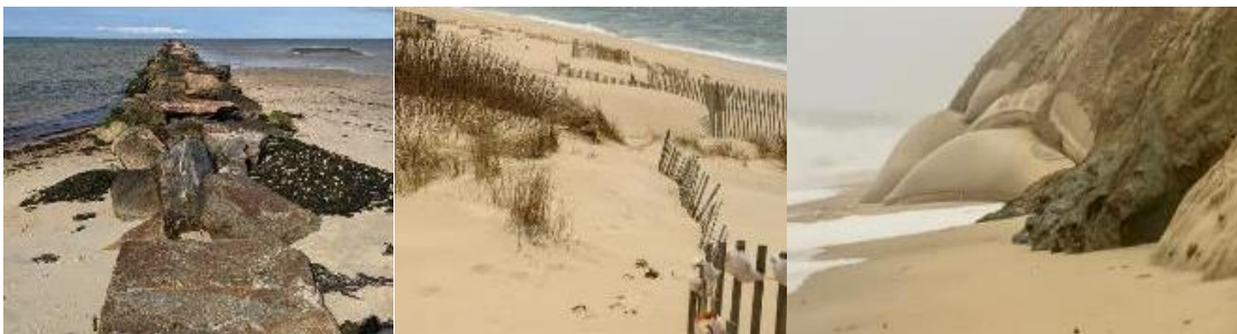
Figure 1. Erosion Control Structures: L: Jetty at Jetties Beach C: Sand fencing and vegetation at Madaket Beach R: Geotubes at Sconset Beach https://www.savenantucketbeaches.org/
