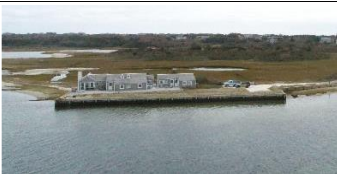
Figure 6. The picture above shows an example of drone photography, courtesy of Burton Balkind. The picture displays a wooden bulkhead installed at a house near Pimney's Point.
