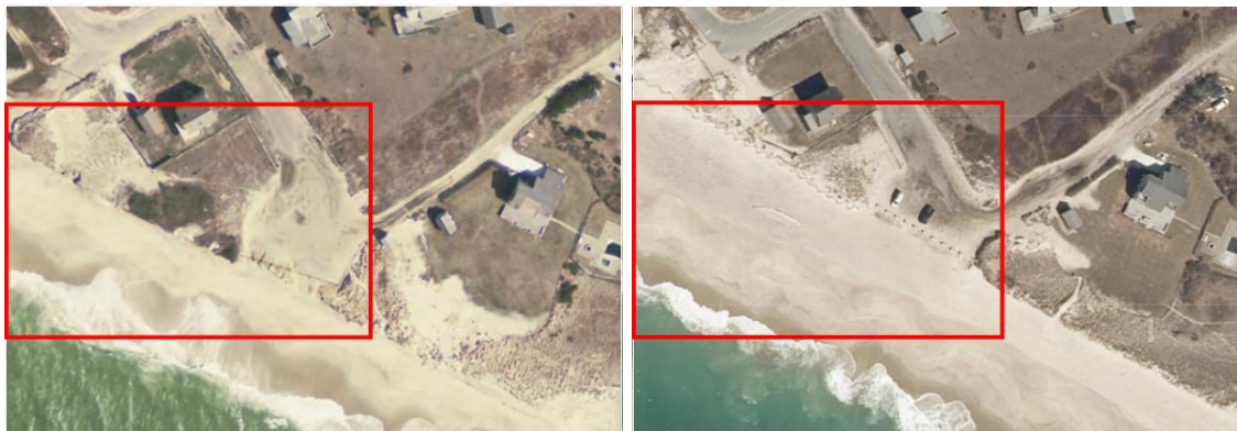
Figure 16. Madaket Beach Parking Lot erosion from MORIS: L: Madaket Beach Parking Lot in 2014 R: Madaket Beach Parking Lot in 2021 https://czm-moris-mass-eoeea.hub.arcgis.com/#DataViewer
