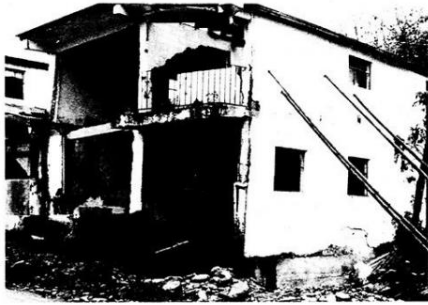
Figure 16. A collapsed building
