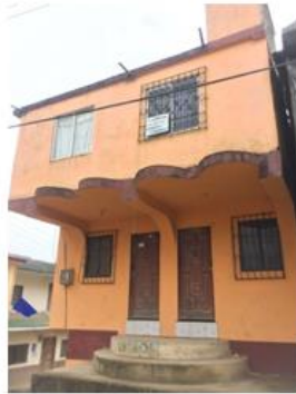
Figure 7. Adobe with concrete façade
