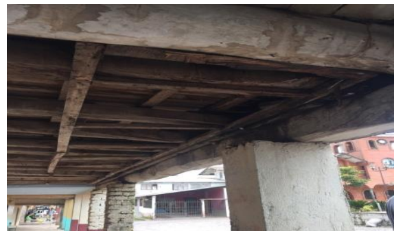
Figure 9. Wooden beams used for support
