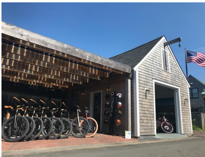
Figure 6. Solar-powered pergola used at Wheels of Delight (E-Bike Sales Rentals, n.d.)
