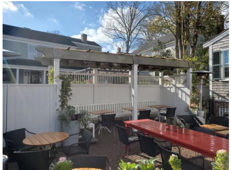
Figure 12. Solar-viable pergola at Corner Table Cafe
