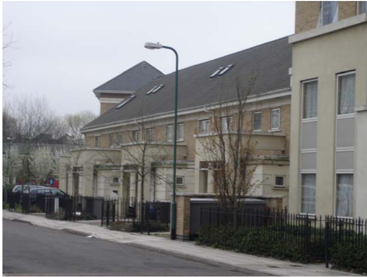
Carlton Vale Development
