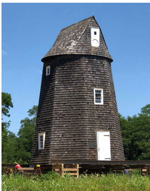
Figure 2.3.2: Raising of the Foundation (Shelter Island Reporter, 2018)
