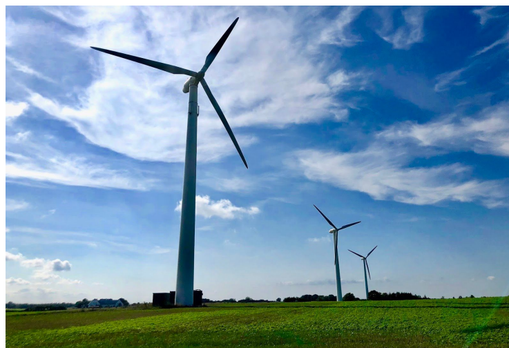
Figure 2.4.1: Modern Wind Turbines (Campbell, 2018)
