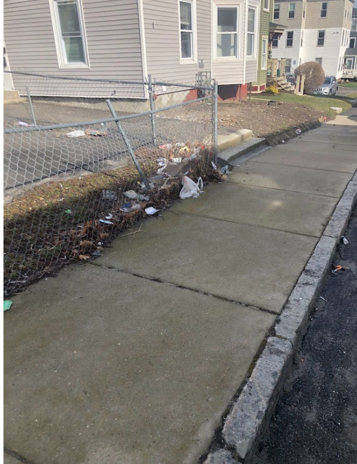
Figure 11: Trash Stuck on a Fence
