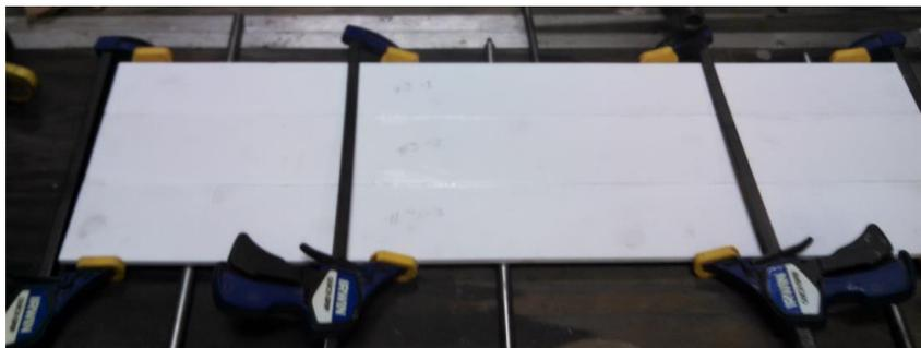
Figure 29: Clamped Tier 1 to Allow Proper Setting Of Biscuit Joints
