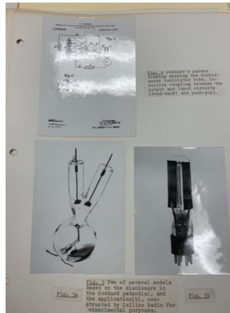
Figure 28: Oscillator Patent Drawing and Models Based on Them (Goddard, 1902-1907)
