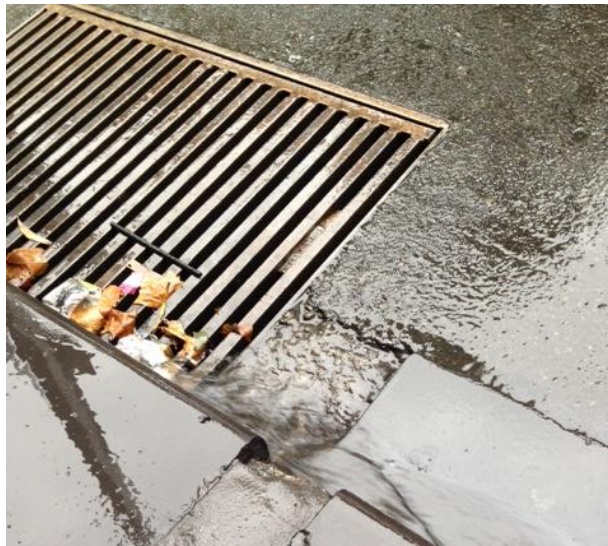
Figure 3: Stormwater drain in Melbourne, AU
