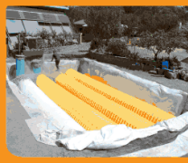
CERES 50,000 litre underground tank
