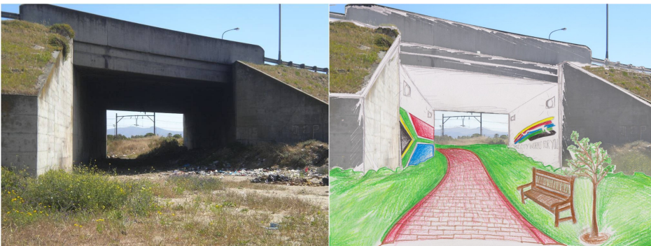
Figure 9: N2 Underpass vision with security lights, pathway, and signed space
