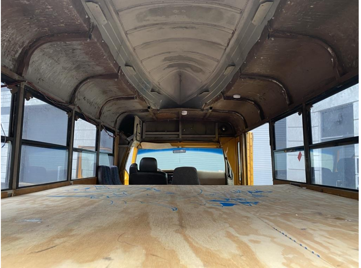
Figure 2, bus 1.5” cubic steel frame and aluminum roof raise
