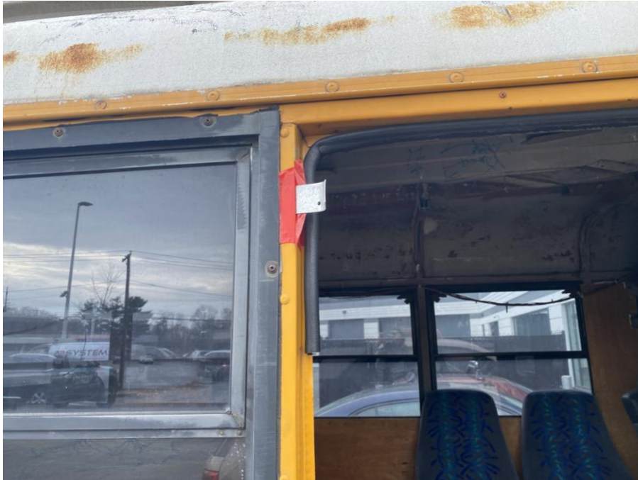
Figure 4, blower door bracket
