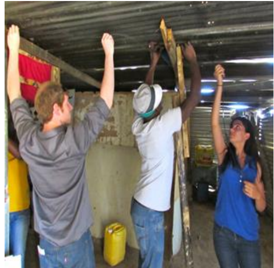
Figure 24: Mounting the Control Box and Setting up the Lights
