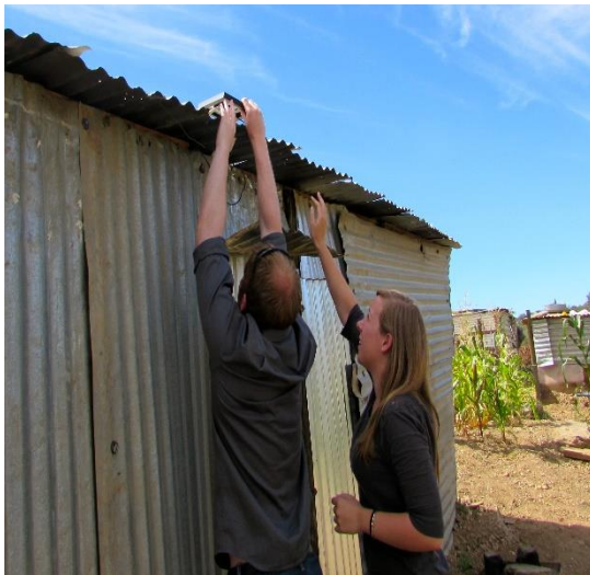
Figure 23: Placing the Solar Panel on the Roof
