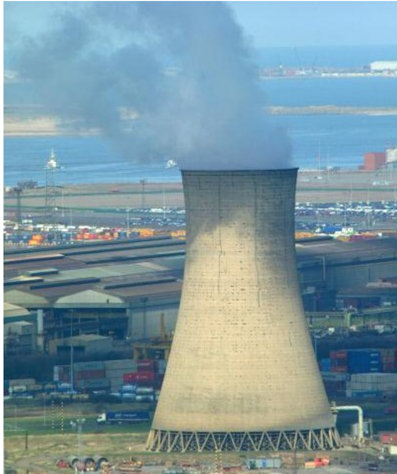
Figure 2.1: Natural Draft Cooling Tower (Britton, I, 2002)
