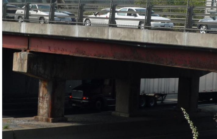
Figure 8: Concrete pier on the Belmont Street/Route 9 Bridge
