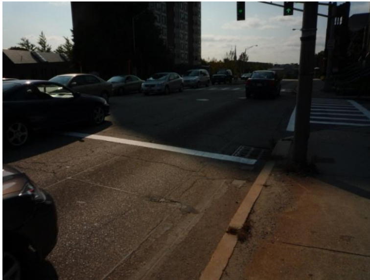
Figure 6: Wearing surface on the Belmont Street/Route 9 highway overpass
