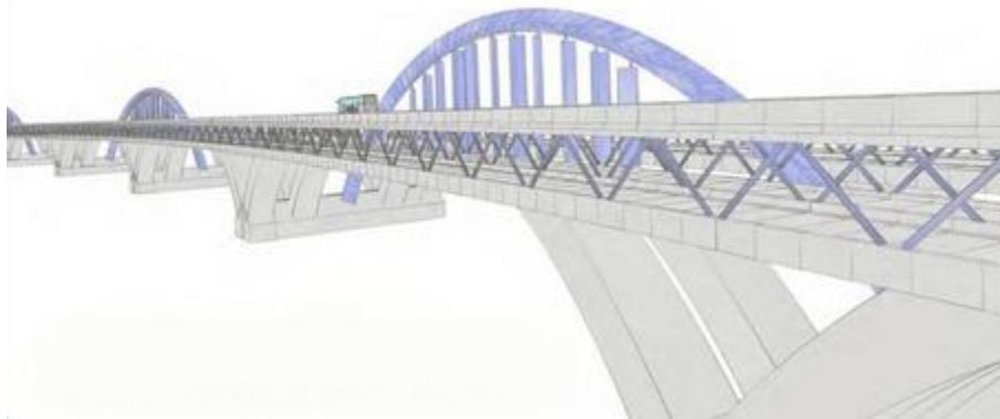
Figure 55: New Interstate 5 bridge crossing over the Columbia River shows vertical wind turbines in blue (taken from http://www.oregonlive.com/environment )
