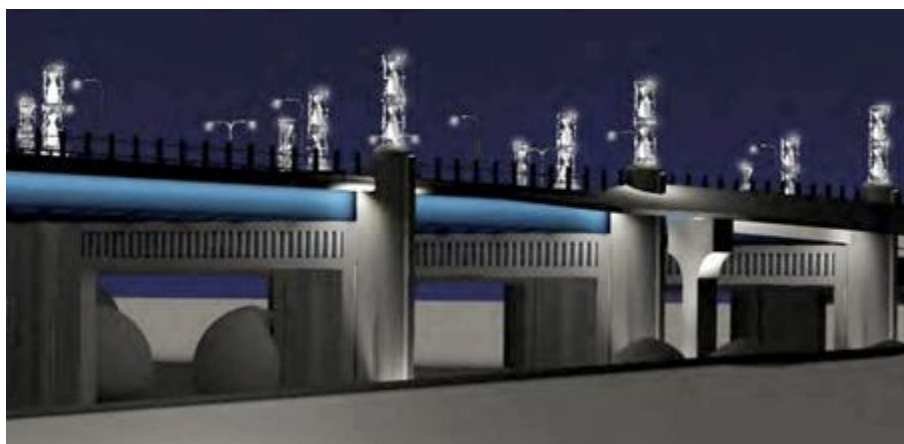
Figure 56: Flat Interstate 5 bridge design with wind turbine mounted along the bridge, similar to a sculpture design (taken from http://www.oregonlive.com/environment )
