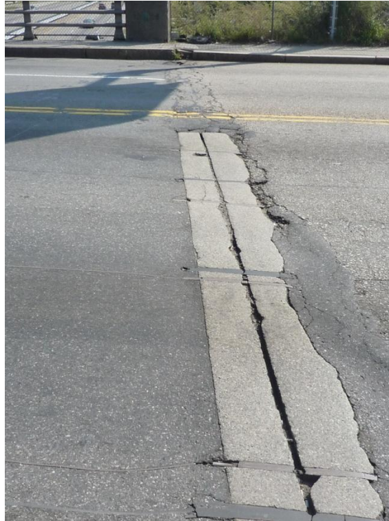
Figure 11: Wearing surface on Belmont Street/Route 9 Bridge
