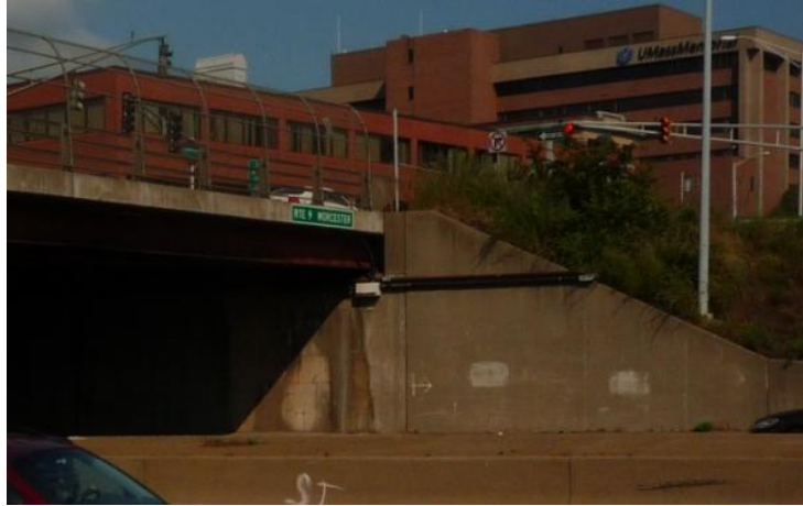
Figure 9: Example of the wingwall and backwall on Belmont Street/Route 9 Bridge
