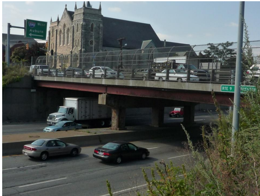
Figure 1: The existing Belmont Street/Route 9 overpass
