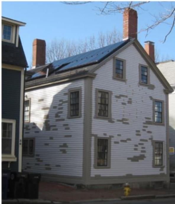
Appropriate installations balance functionality with aesthetics and minimize the appearance of solar panels through color, placement, and continuity of the roof plane.
